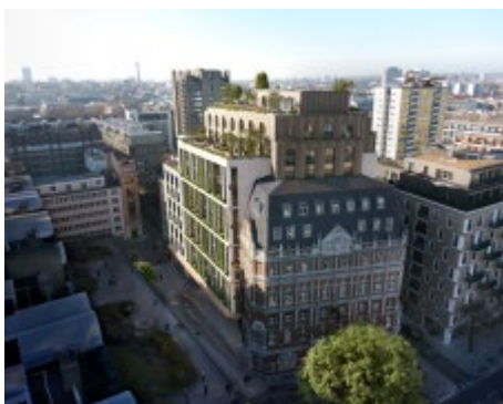
CGI of completed UNO development
